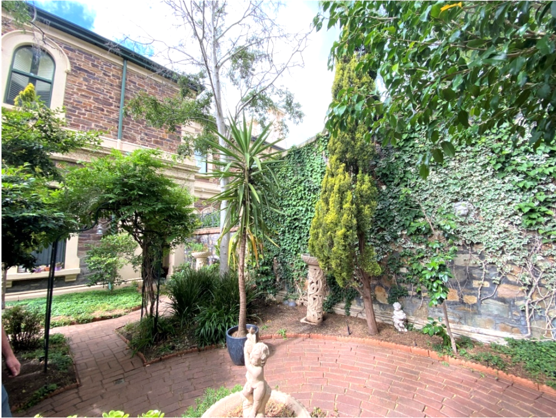
Figure 3.5 - view of courtyard at 18 Dimora Court with west wall of subject garage
